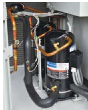
Partial view of the refrigeration circuit
